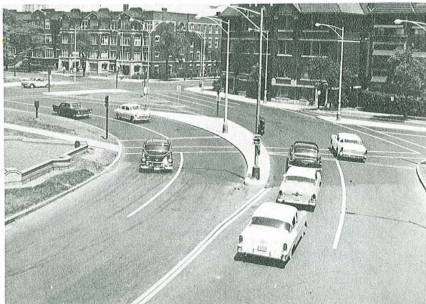
Figure 4-23. Channelization, signalization, and pavement markings are used to control movement within this intersection. The islands also serve as pedestrian refuge islands.
