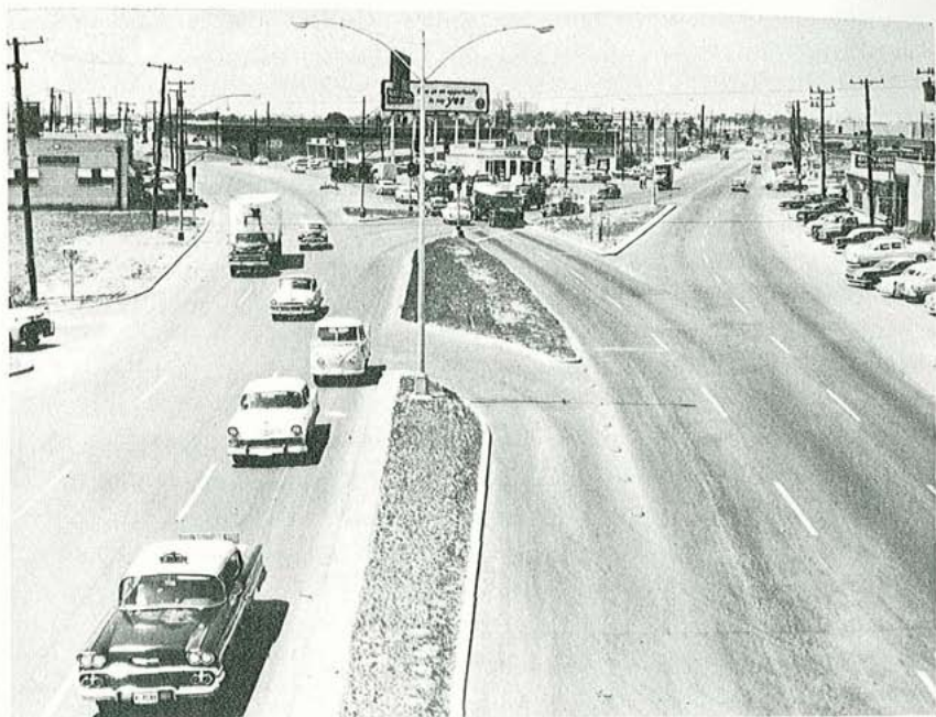
Figure 4-3. Channelizing islands at a signalized Y-intersection. Concrete curbs delineate the island edges. Mushroom buttons separate a left-turn lane from the through lanes.
