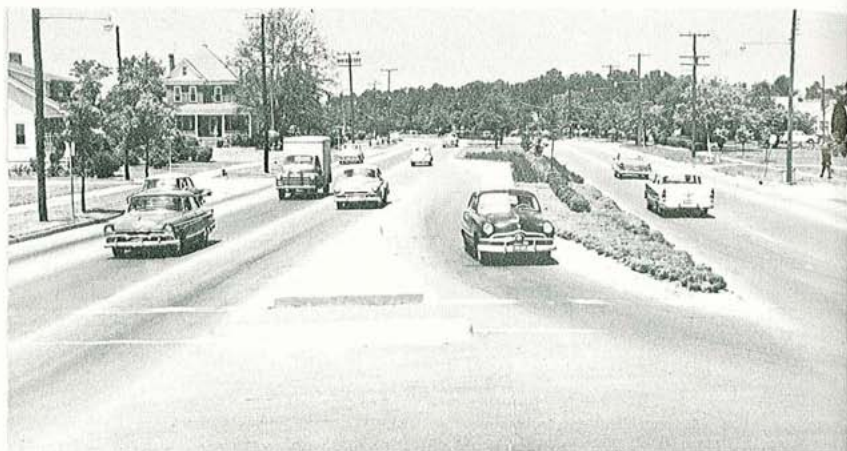
Figure 4-5. Walk-through pedestrian refuge island that also serves to separate a median lane from the through lanes. Approach-end treatment consists of pavement markings and high-visibility painted curb.
