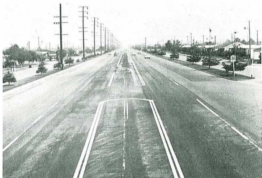
Figure 4-12. Expressway with a painted-line median and frontage roads. The divisional island or outer separator is sodded and planted, and outlined by vertical curb.
