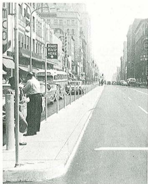
Figure 4-9. Mid-street bus loading platform of concrete. Steel posts and chains provide side protection and discourage mid-block crossings by pedestrians. End protection is provided by heavy steel post and painted curb.
