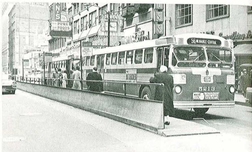
Figure 4-8. Mid-street bus loading platform on a one-way street. The loading area is composed of wood plank deck, and is protected by sheet metal splash plate. Advance warning is given by signs at end facing traffic.
