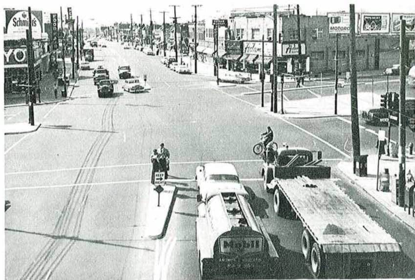
Figure 4-6. Pedestrian refuge island with raised platform ending at crosswalk line. Approach-end treatment consists of pavement markings, reflectorized sign, and hazard marker.
