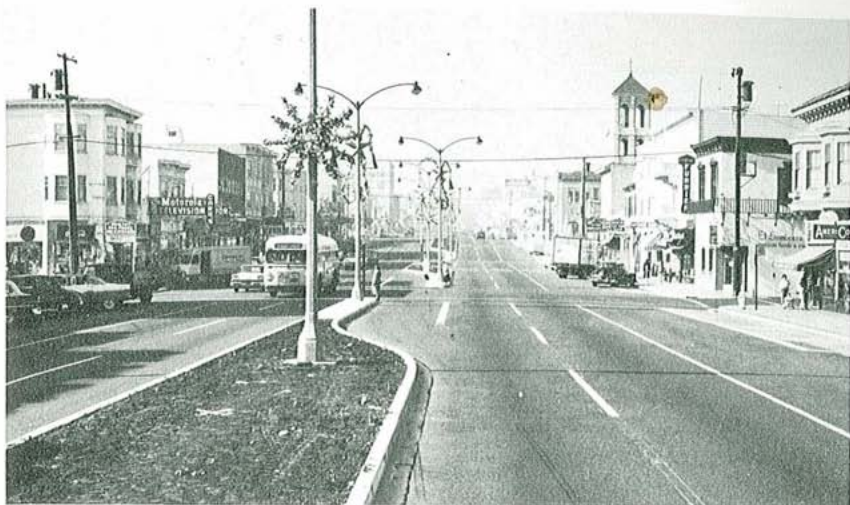
Figure 4-14. Separate left-turn lanes are notched into a relatively wide earth-filled median outlined with vertical curbs. The median lane separator is paved with concrete to serve as a pedestrian island.
