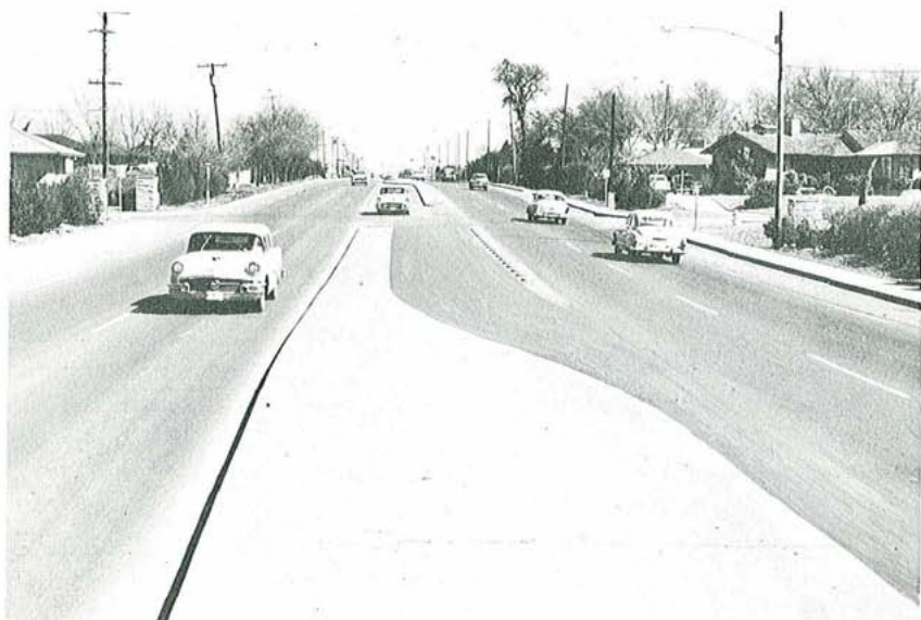
Figure 4-10. Concrete median on a major street in a residential area. Median lanes are provided for storage and safety at intersections. Mushroom buttons separate the left-turn lanes from the through lanes.
