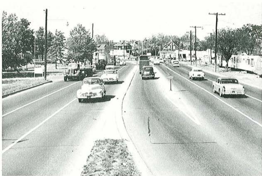
Figure 4-13. Median lane with mountable concrete curb traffic separators having a scored face for light reflection. Pavement markings and a hazard marker give advance warning of the introduced separator.
