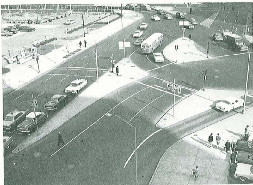
Figure 4-21. Channelization is accomplished through use of both concrete and painted islands in this intersection. The entire area is well illuminated.
