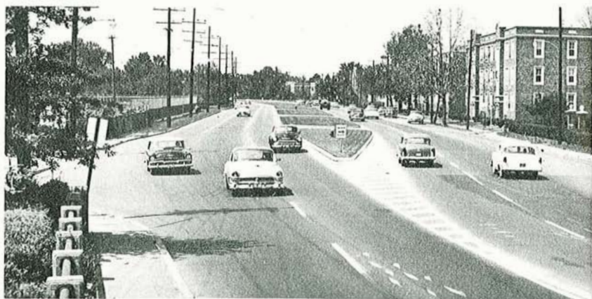
Figure 4-2. Turf median outlined by a mountable curb in a suburban area. Approach-end treatment consists of painted lines on the pavement, painted curb, and a reflectorized sign.
