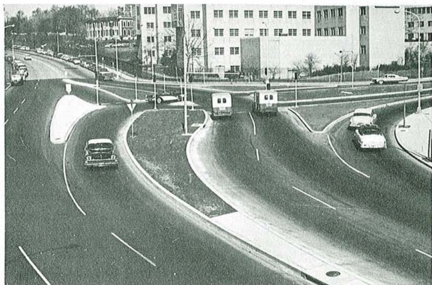
Figure 4-22. The smaller islands of this channelized intersection are of concrete, and the larger are of earth with concrete curb delineation.
