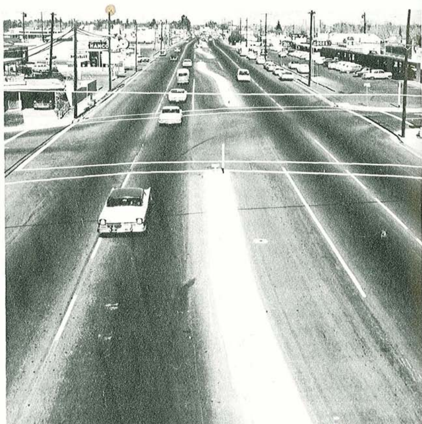
Figure 4-15. Raised concrete median warped to provide protection and storage for left-turning vehicles at intersections. Painted curbs and hazard markers mark the islands.
