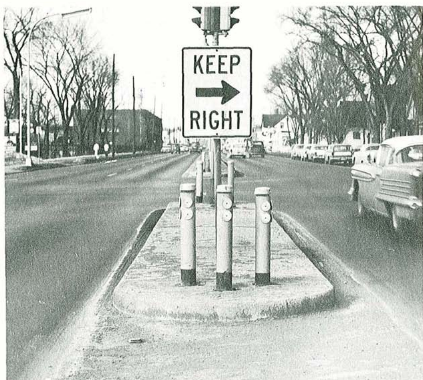
Figure 4-7. Pedestrian refuge island protected by a barrier of steel posts. The reflectorized sign and the reflectors on the posts give advance warning of the island.
