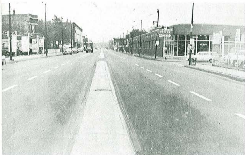
Figure 4-16. Low divisional island that can be crossed by vehicles but which discourages mid-block left turns.
