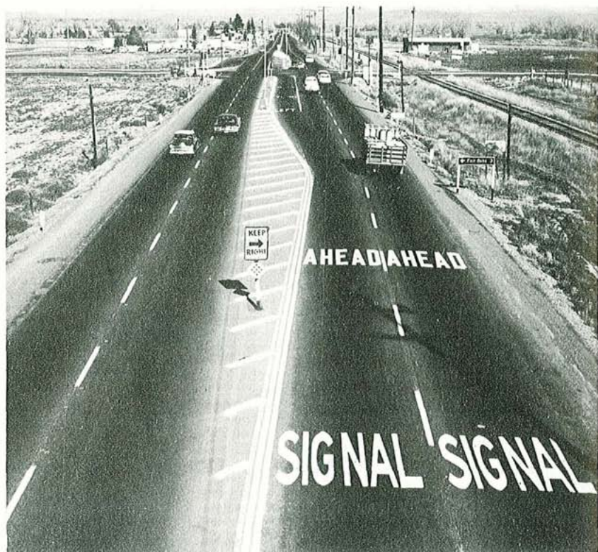
Figure 4-11. Divisional island of raised bars introduced to provide a left-turn lane. The island at the intersection is delineated by mountable curb and is illuminated. Included in the approach-end treatment are a reflectorized sign and a hazard marker.
