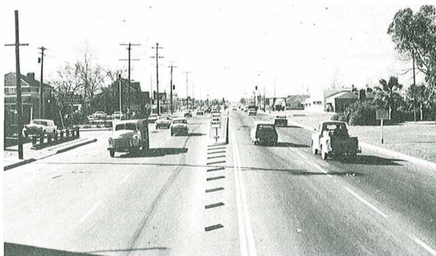
Figure 4-4. The transition from a 4-lane undivided roadway to a 4-lane highway with a curbed median is effected through the use of raised concrete bars and pavement markings. Further warning is given by the use of a sign, a hazard marker, and a high-visibility curb.
