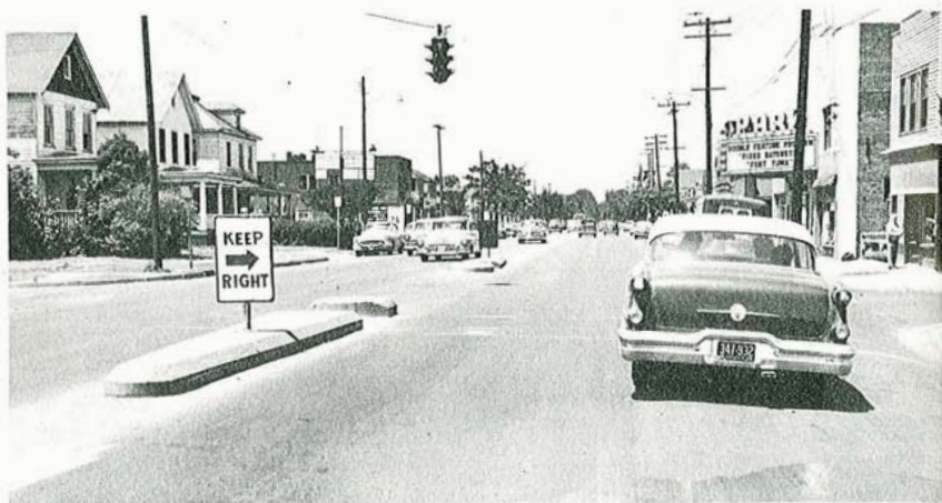
Figure 4-1. Pedestrian refuge island with walk-through crosswalk. Approach-end treatment consists of pavement markings and a reflectorized sign.
