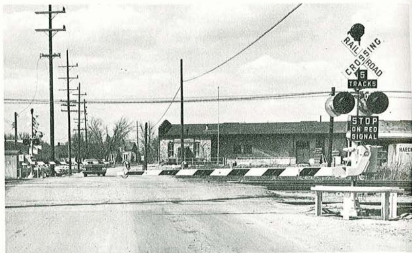
Figure 3-6. Train-approach signal installations at railroad-highway grade crossings.
