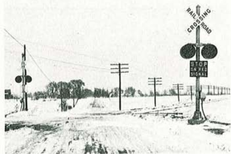
Figure 3-6. Train-approach signal installations at railroad-highway grade crossings.
